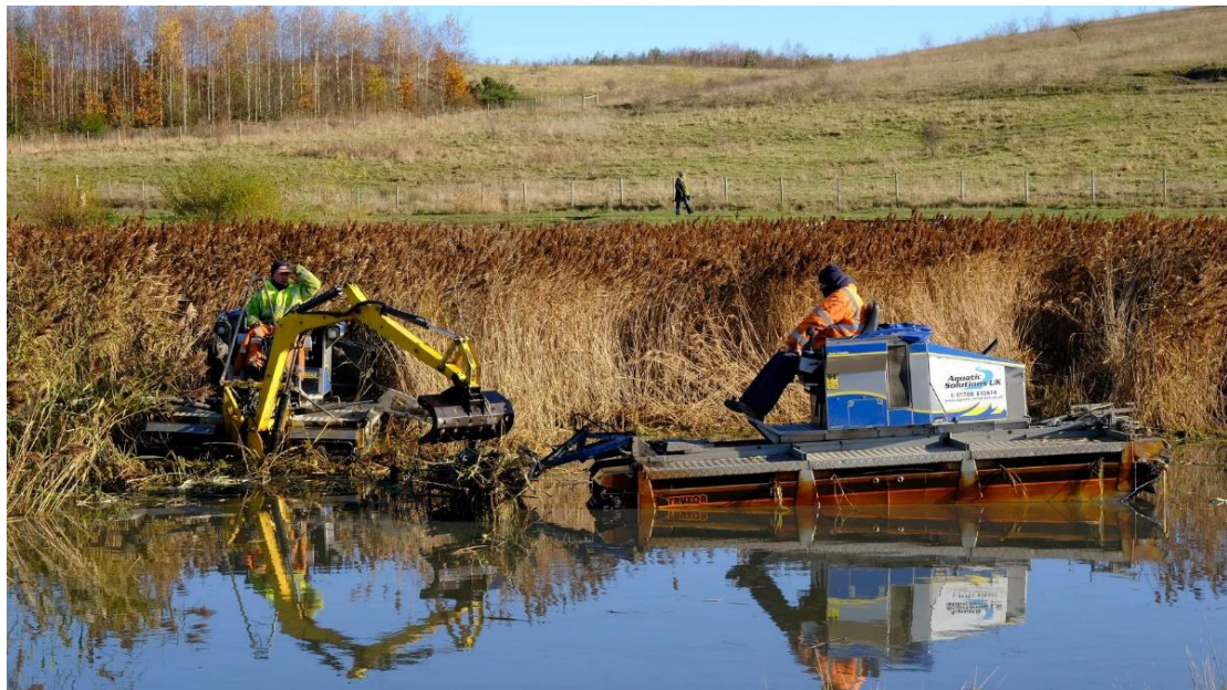
Reed removal using amphibious equipment on the Central Lagoon
